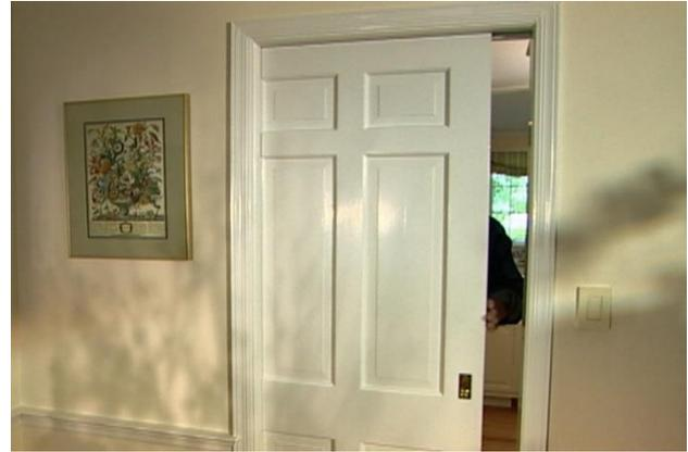
Will light switches, outlets, temperature controls, alarm key pad, etc., need to be relocated in order to allow room for the barn door or pocket to operate? If so, be sure to relocate in an accessible area.
