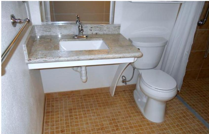
Wall hung counter top with sink. This design does not provide any storage under the counter top.
