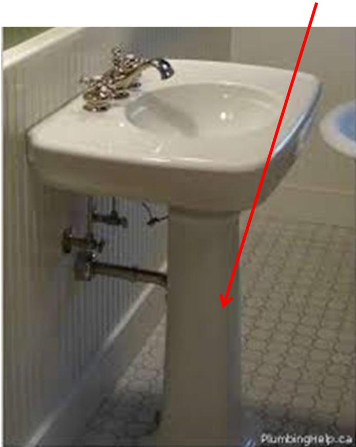
When removing or modifying an existing base cabinet/vanity, the floor covering will need to be addressed. Typically, these fixtures are installed prior to the floor covering so when they are removed/modified, the floor space once occupied by the base cabinet/vanity will not be covered by the floor covering. The wall covering may also need to be addressed.
