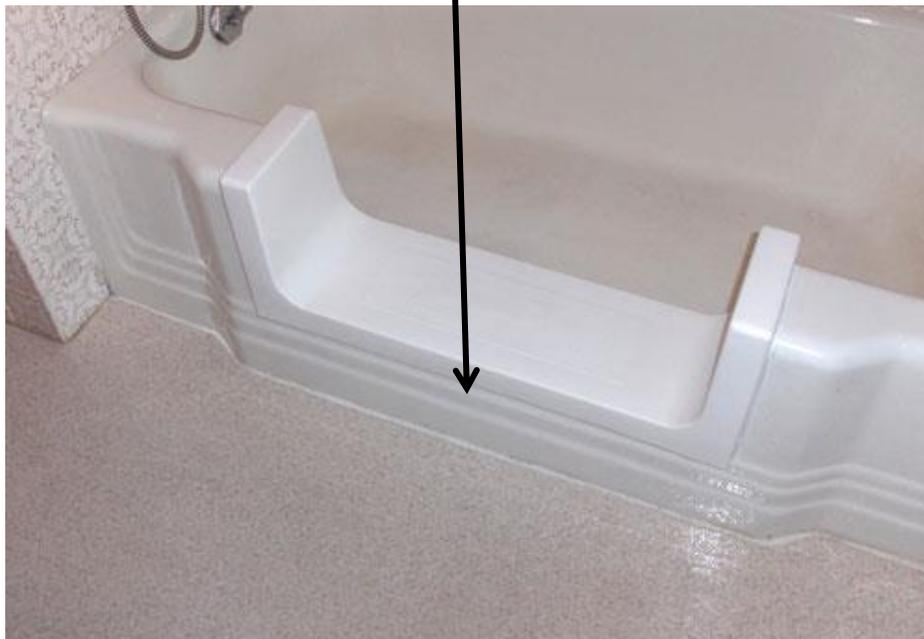
A tub cut can also be used when an accessible shower is needed but it is not possible to install either a roll in shower or a walk in shower.
